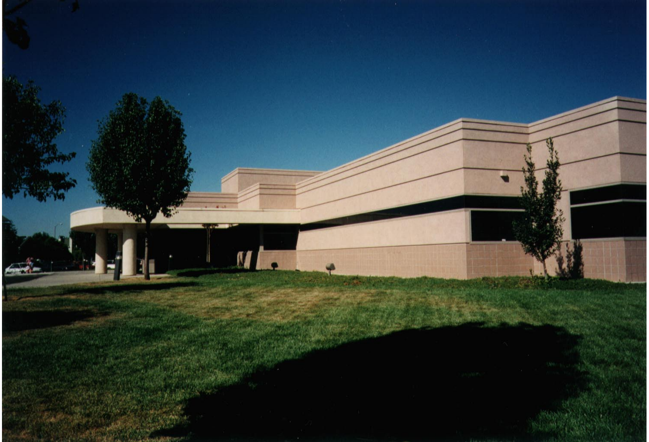
Figure 1(a): Ground-level view of the Davis building
