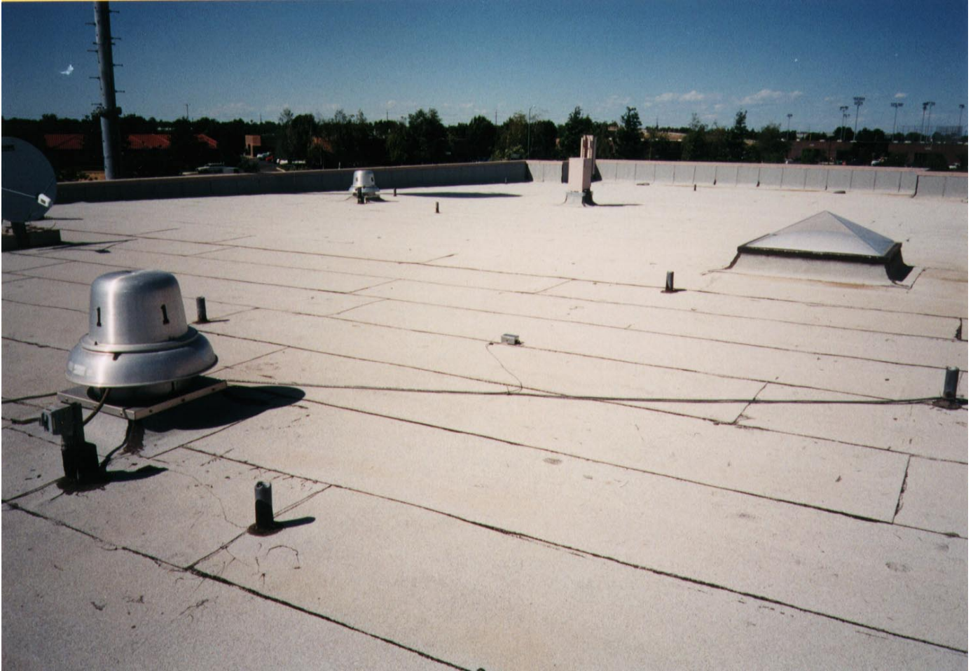
Figure 1(b): Roof of the Davis building.
